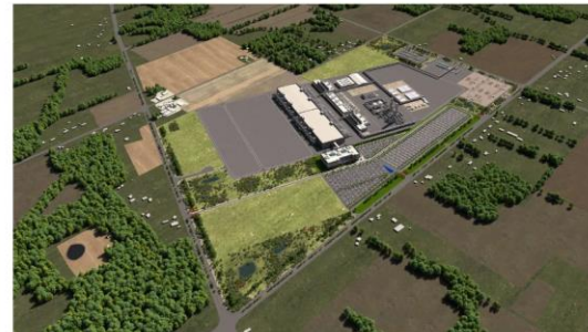
A rendering of two Intel computer chip factories that are scheduled to open by 2025. Intel
